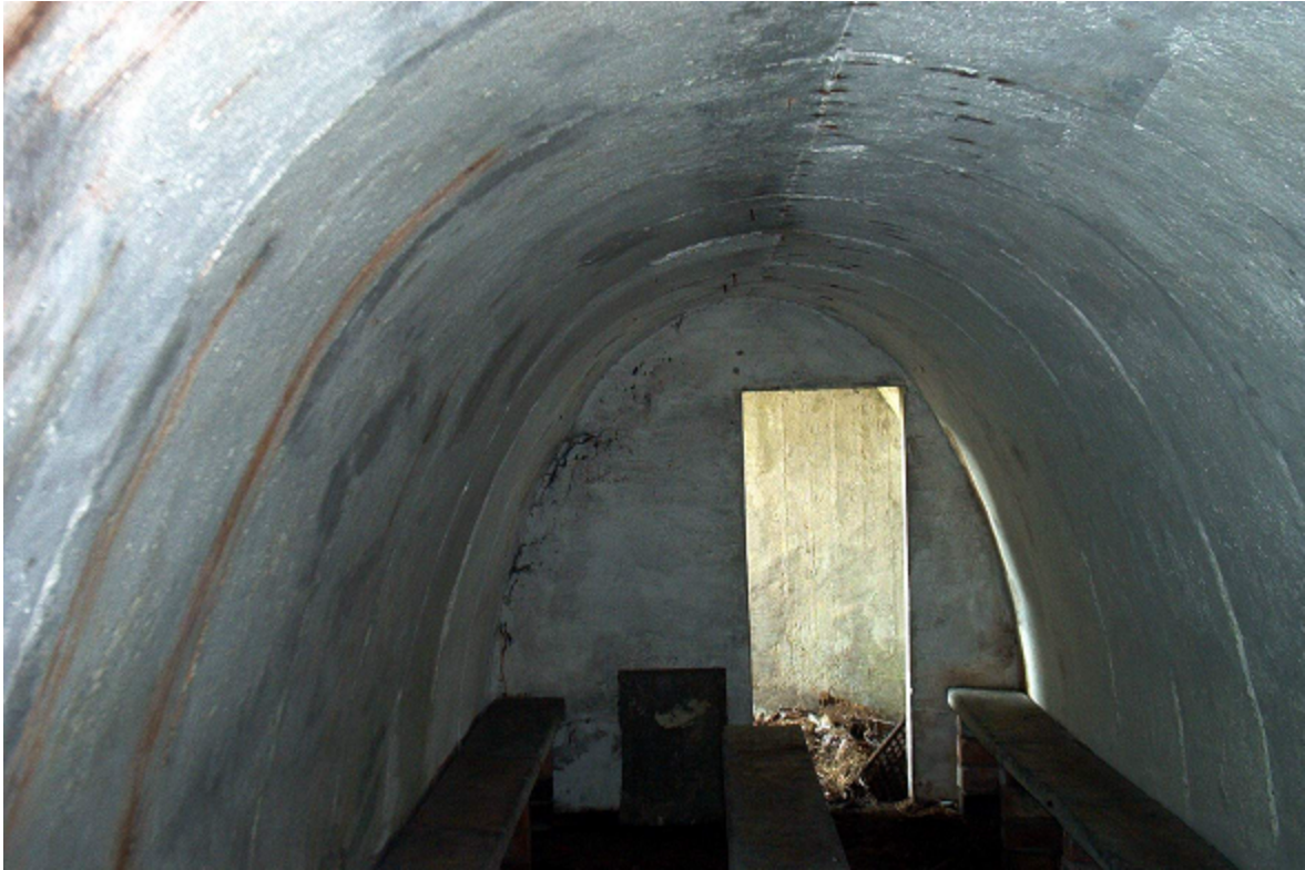
Figure 3 Interior of Shelter 3 showing staples in the ceiling
