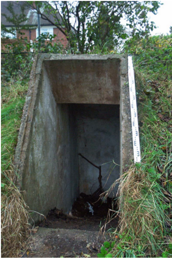
Figure 1 Entrance to Air Raid Shelter
