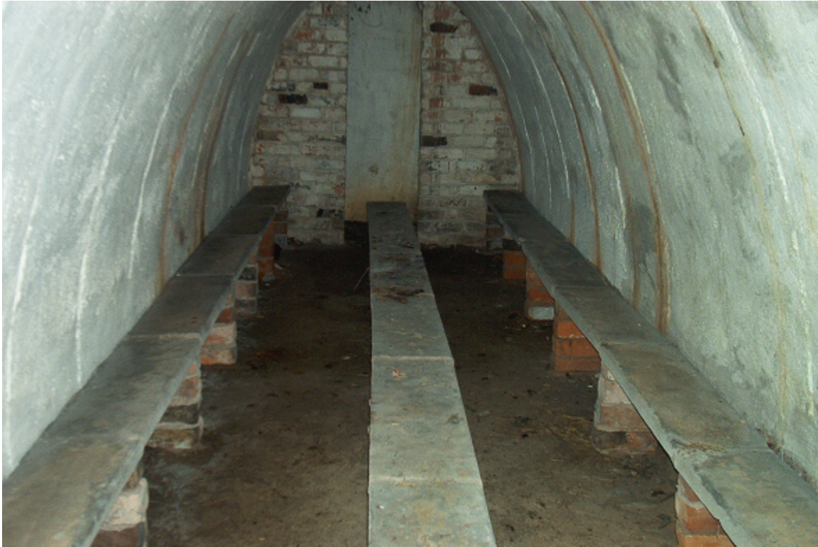
Figure 6 Typical interior of an Air Raid Shelter
