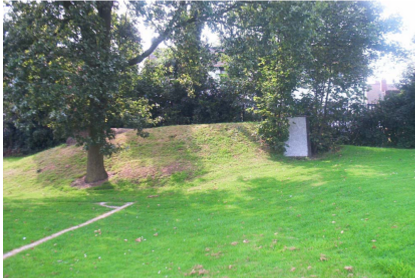
Figure 10 General view of the Air Raid Shelter at St Luke's.
